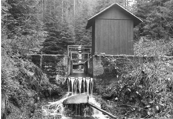
Figure 14. View of the limnigraph station on the CE-B sub-watershed
