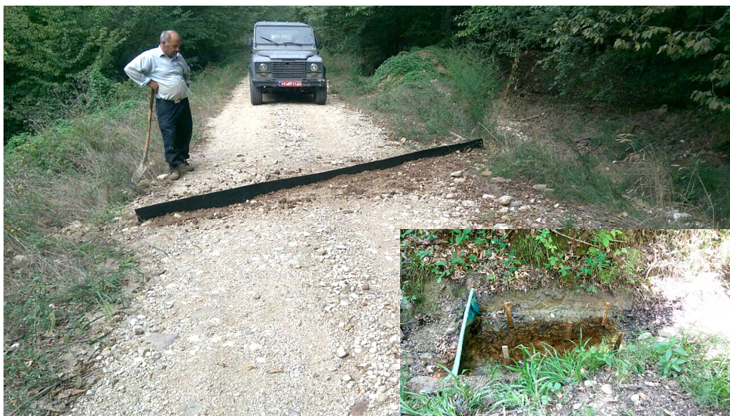
Figure 2. Rubber bar for diverting runoff into a sediment trap
